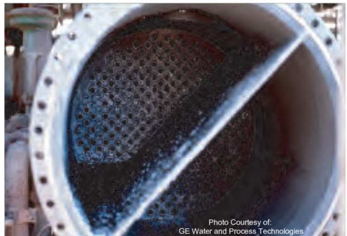
Figure 6. Soft Coke Precipitation Fouling
